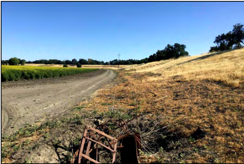
Photo 3. View of the land side of the west ridge cut levee, view northeast, 05/20/2021.
