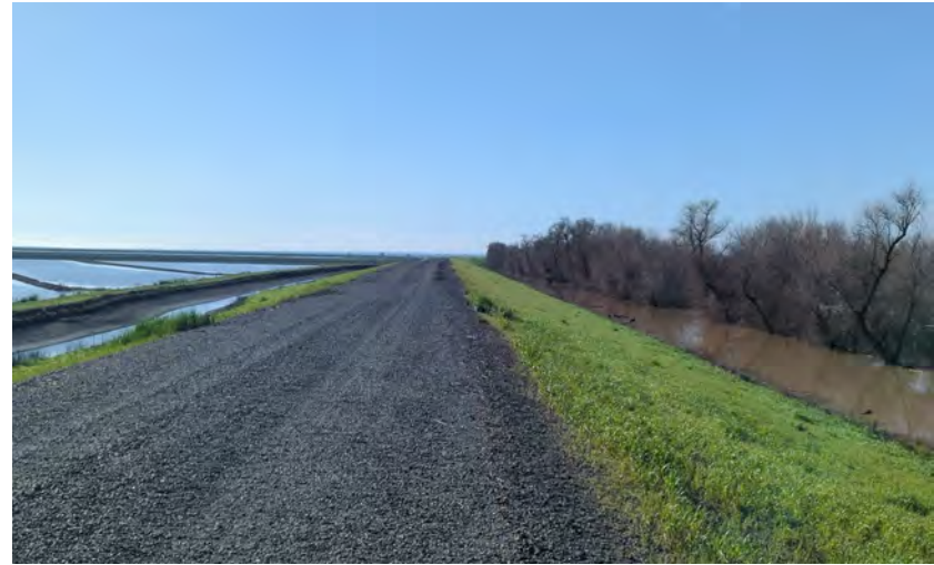
Representative photo of top of levee, facing southeast.. Photo taken February 22, 2024.
