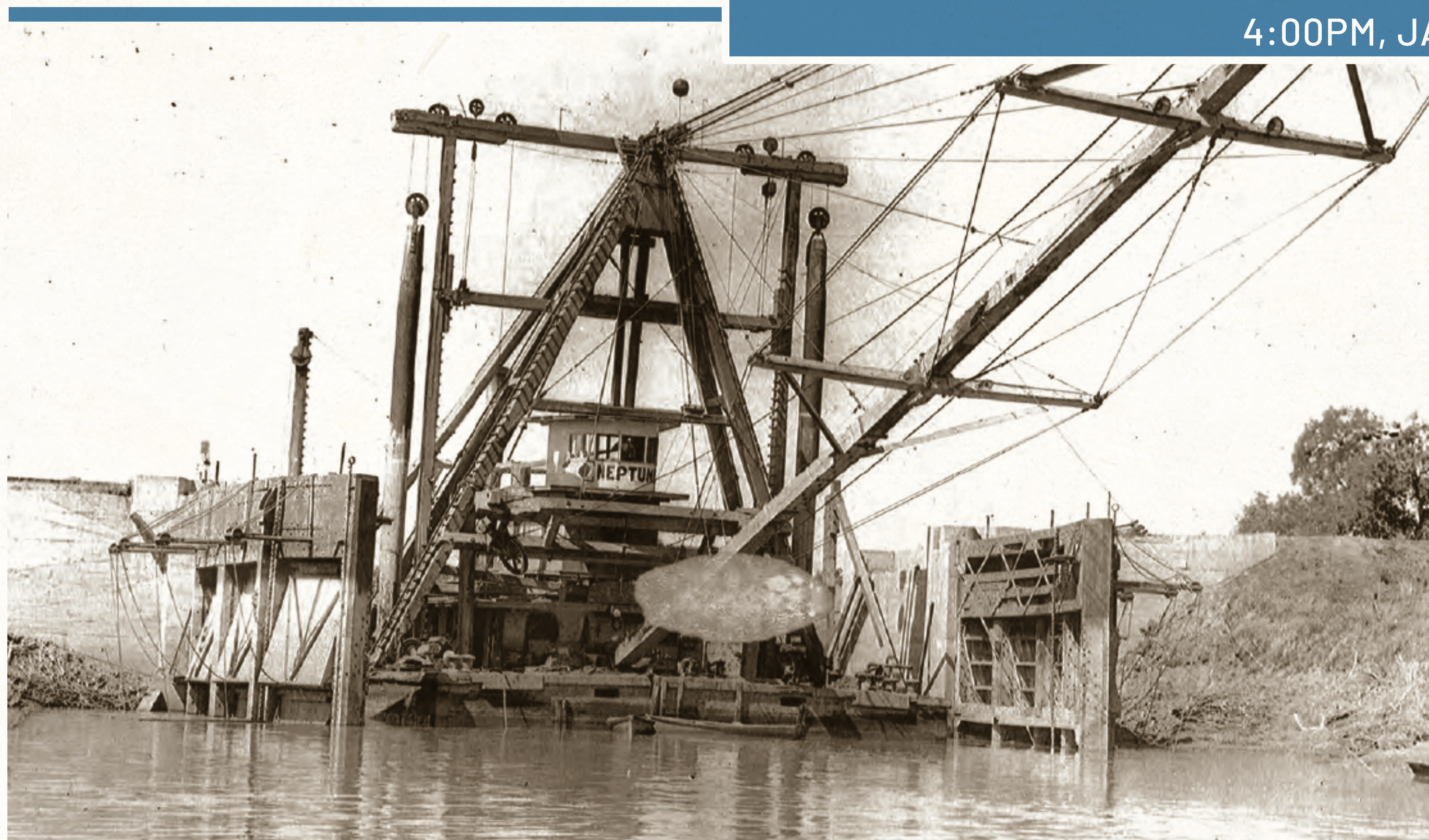
DREDGER "NEPTUNE" PASSES THROUGH THE OUTFALL GATES NEAR KNIGHTS LANDING ENTERING THE RIVER. JUNE 1917
