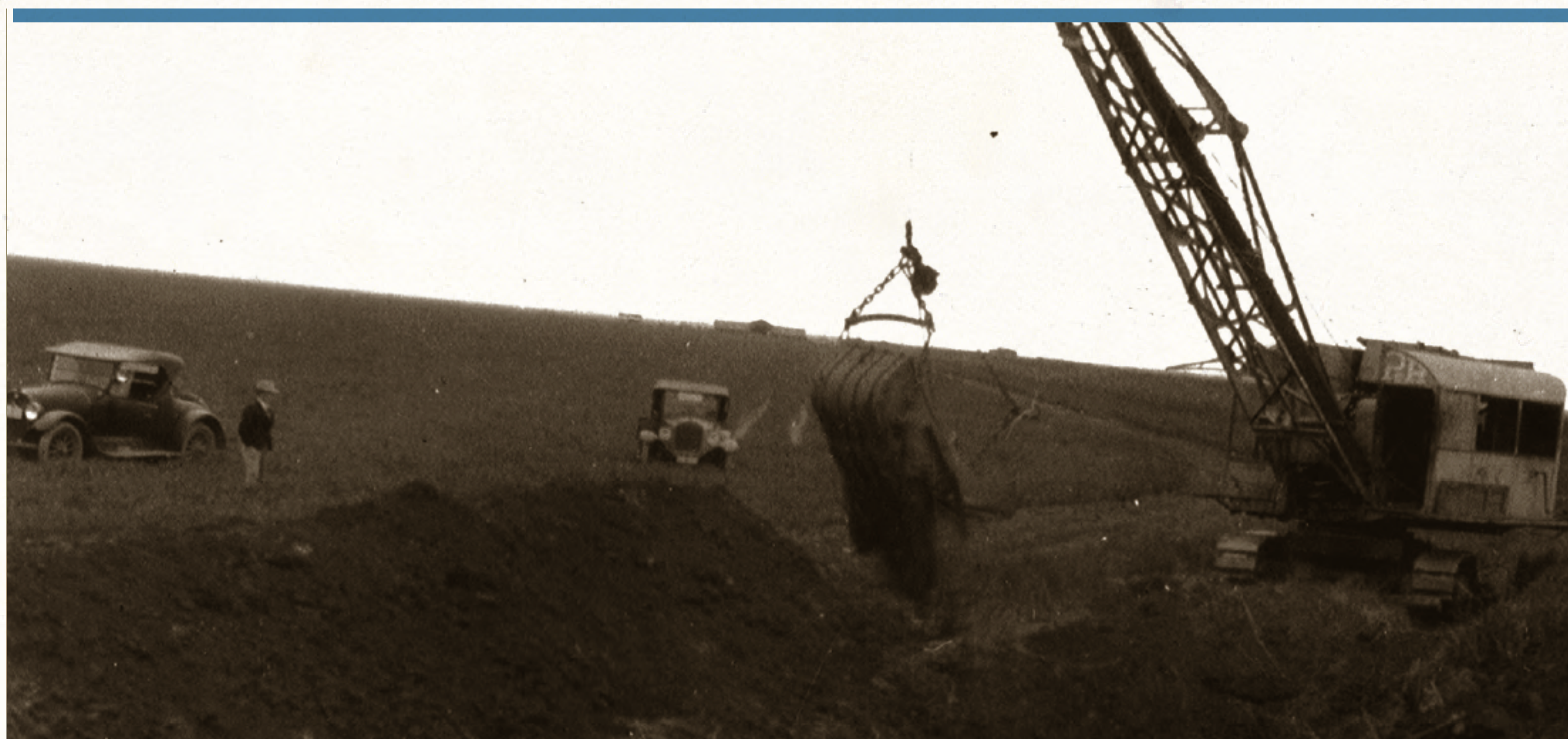
IRRIGATION LATERAL UNDER CONSTRUCTION THROUGH BROWNING RANCH. APRIL 2, 1926
