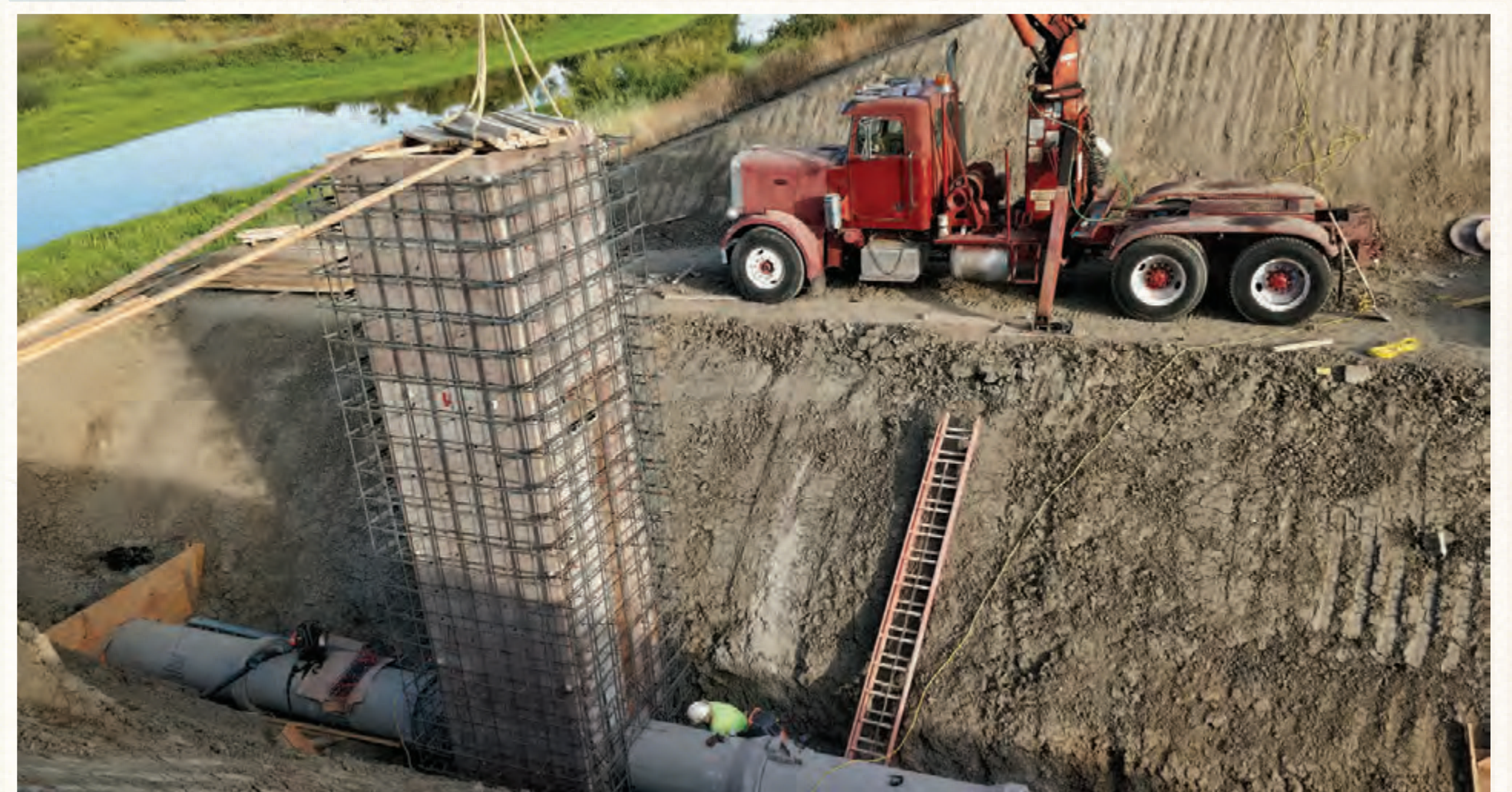
PIPE REPLACEMENT KNIGHTS LANDING RIDGE CUT 2019
