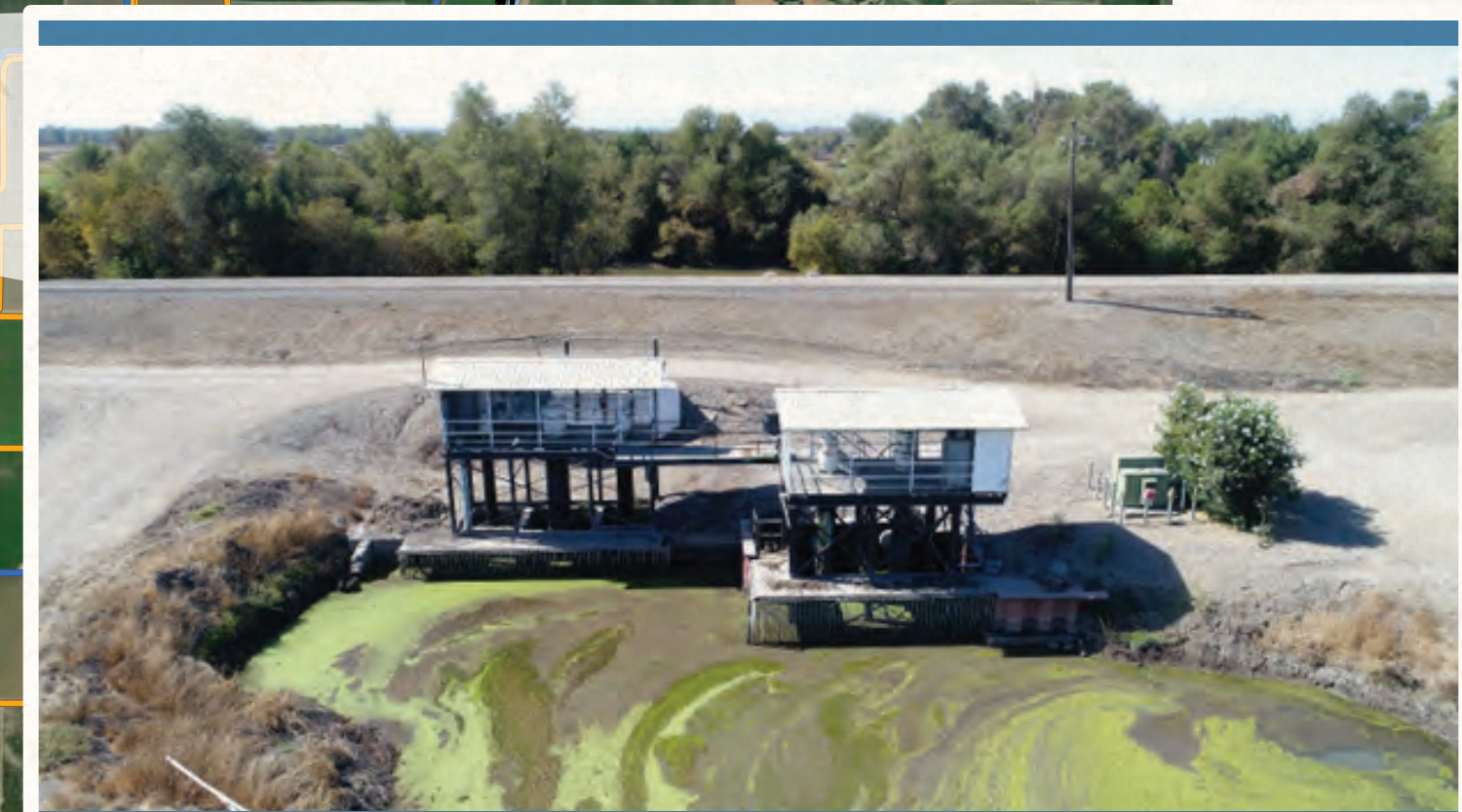
RIGGS RANCH A three-way box system allows for discharge or reuse of drain water, as well as diversion from the Colusa Basin Drain.
