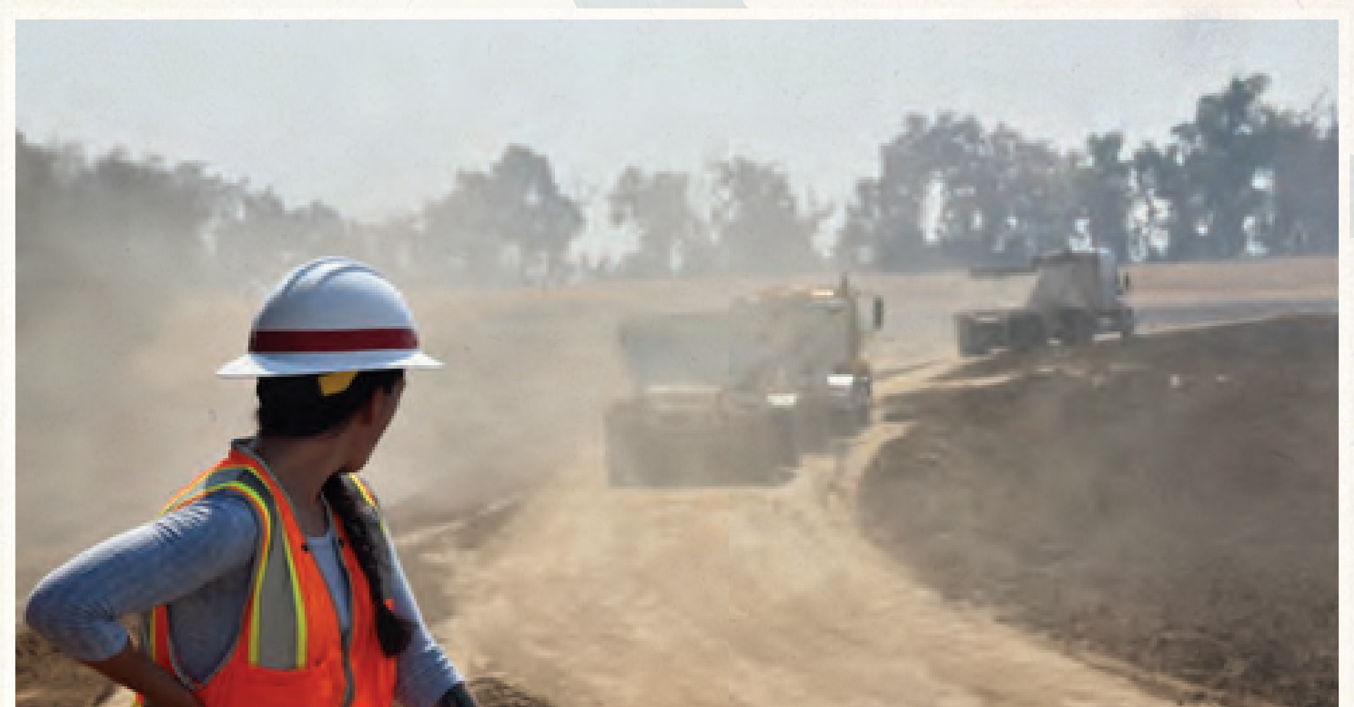
SETBACK LEVEE UPSTREAM OF KNIGHTS LANDING, 2022
