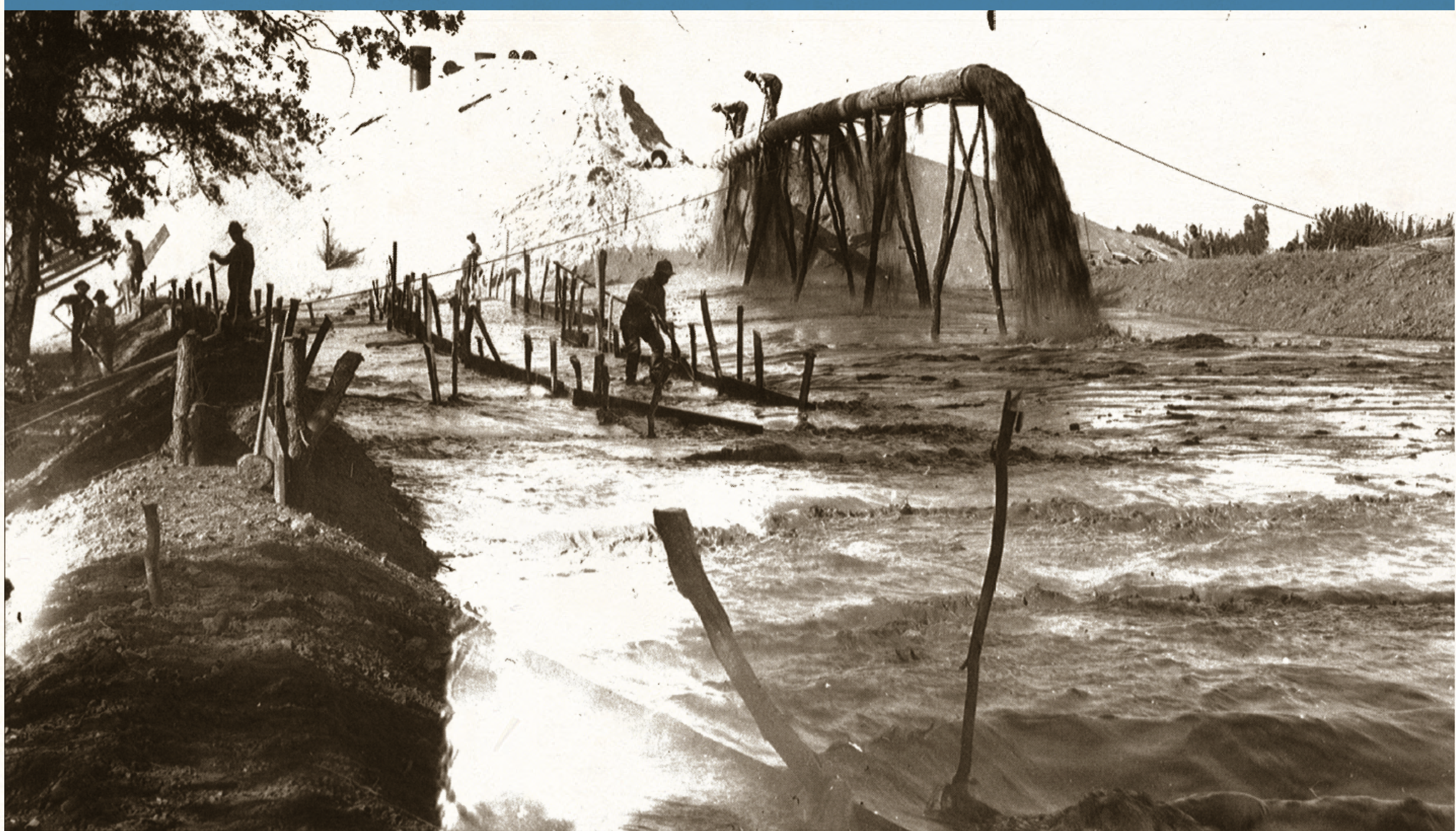
LEVEE CONSTRUCTION WITH SUCTION DREDGE "NATOMAS" OPPOSITE MINISTERIAL BEND. SEPTEMBER 26, 1915
