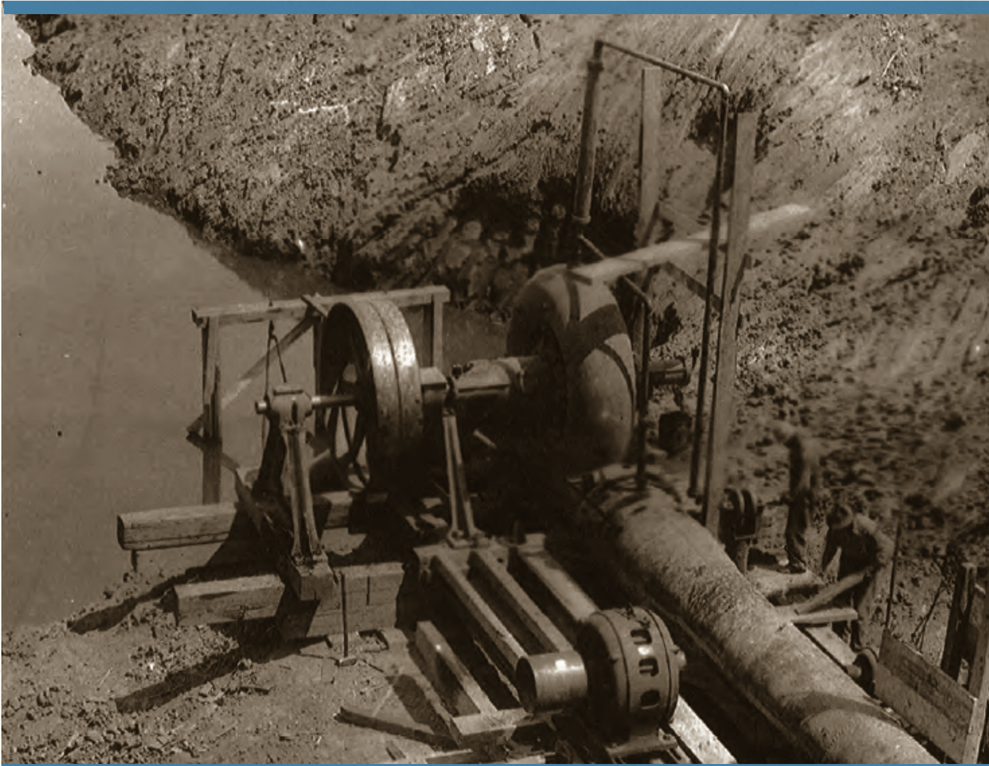
INITIAL TEMPORARY PUMPING PLANT AT WILKINS SLOUGH. JULY 21, 1918
