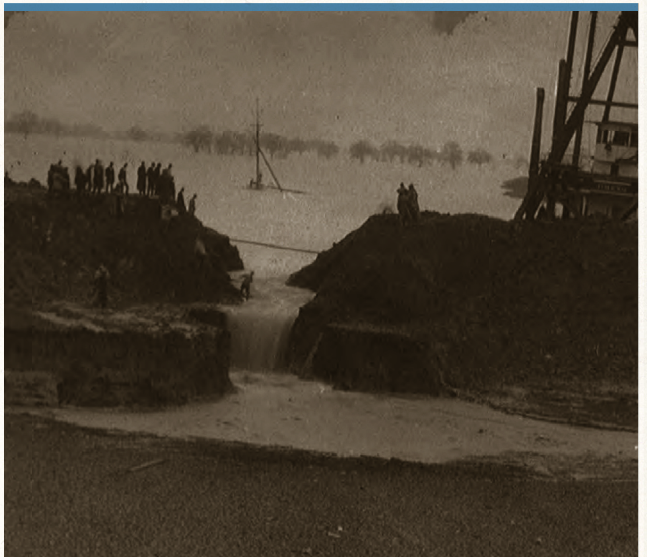
OPENING UP DAM AT HEAD OF RIDGE CUT-ABOVE 50-100 SEC. FT. FLOWING THROUGH. 11:00AM, FEBRUARY 22, 1915
