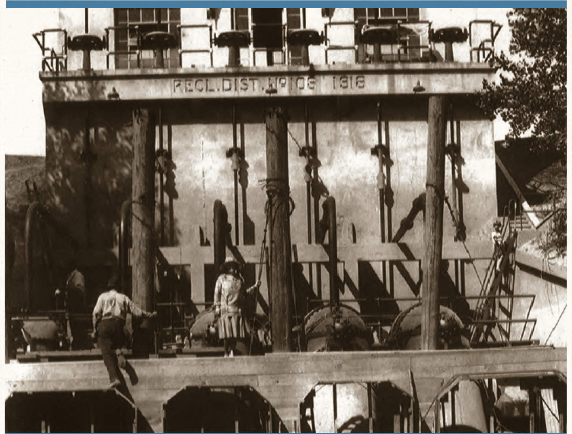
WILKINS SLOUGH PUMPING PLANT INTAKE SUCTION PIPES AND GATES. AUGUST 12, 1927
